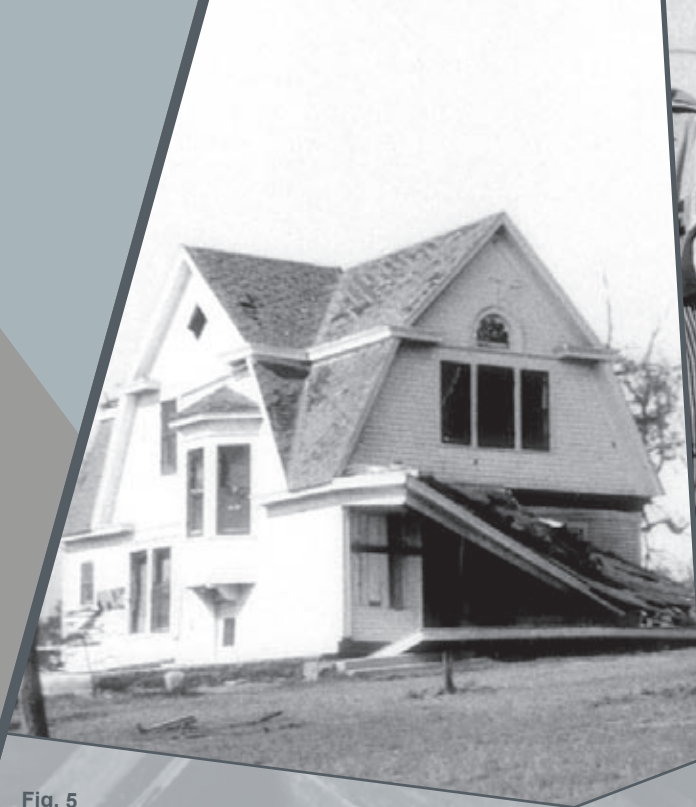
Fig. 5 This two-story home on East Furguson Avenue in Blackwell was damaged by the tornado that devastated eastern portions of the city. Photo courtesy of the Blackwell Journal-Tribune.
