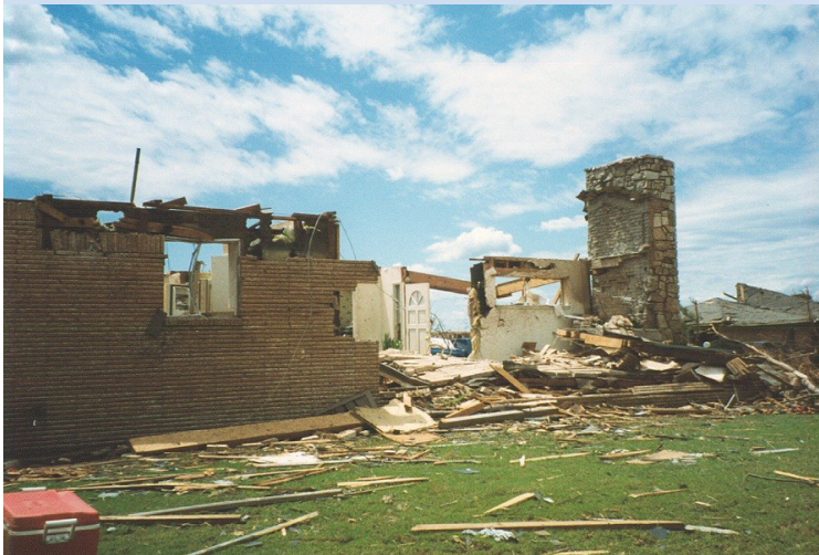
May 3, 1999 Damage in Northeastern Moore (Mike Branick, National Weather Service)
