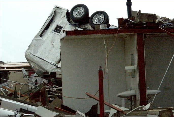
May 4, 2007 Main Street Damage in Greensburg, KS (Nicole Giuliano)
