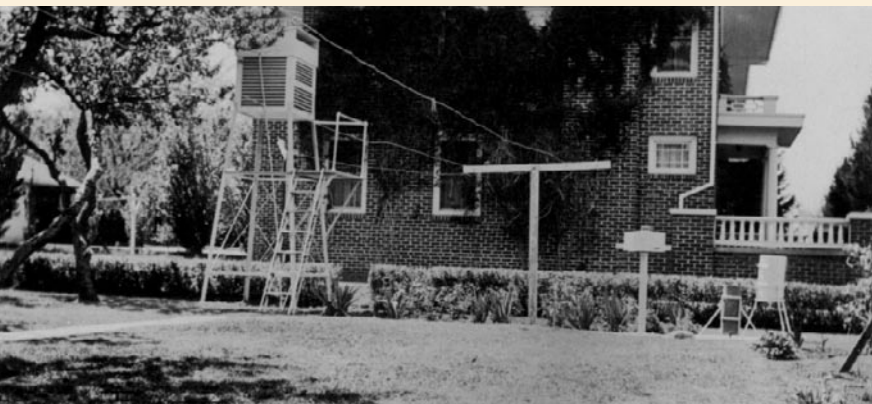
The building's dual role of observatory and residence shows in this picture from April 1934. The south side of the building features a nephoscope (a device that measures cloud movement), rain gauge, snow gauge, instrument shelter and a clothesline for drying the Wahlgren family wardrobe. Photo courtesy of NOAA/NESDIS.
