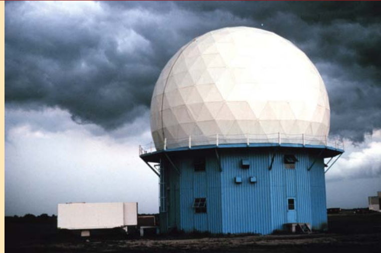
NSSL’s Norman Doppler radar in June 1973, just a few weeks after the Union City tornado. The radar was operated from within the blue building housing the unit. Photo courtesy NOAA Photo Library, NSSL collection.
