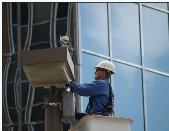
Figure 2a. A Micronet technician deploys the KCB104 traffic light station on 8 May 2008.
